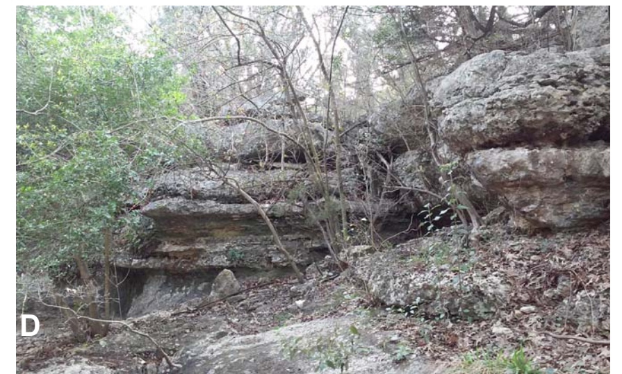
D Deep erosion in channel nearing 20 feet high.
