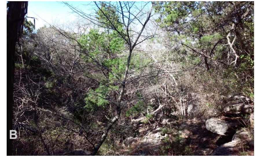
B View of heavy erosion near the top of channel 2.
